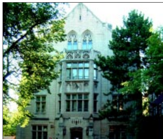
Dolphin System Application: Yale University Music Center (Cooling Tower)
