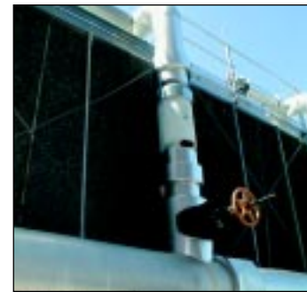
Dolphin System Cooling Tower Project
