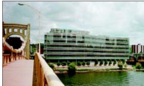
Dolphin System Application: Alcoa Corporate Center (Cooling Towers and Boiler Domestic Hot Water)
