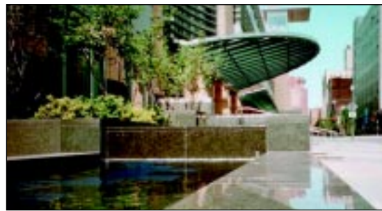
Dolphin System Application: PNC Firstside Banking & Data Processing Center (Cooling Tower and Fountain)
