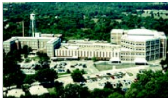
Dolphin System Application: Veterans Affairs Medical Center (Cooling Towers and Steam Boilers)
